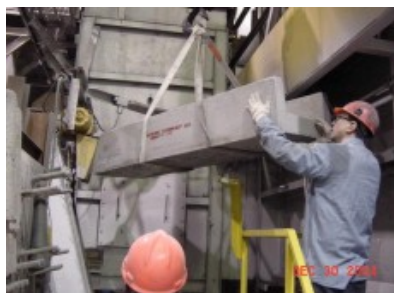
Trough Installation
