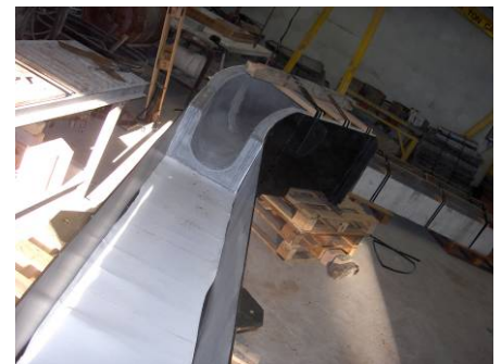
Assembly of Sections
