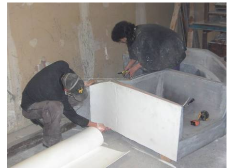
Prepping for Installation
