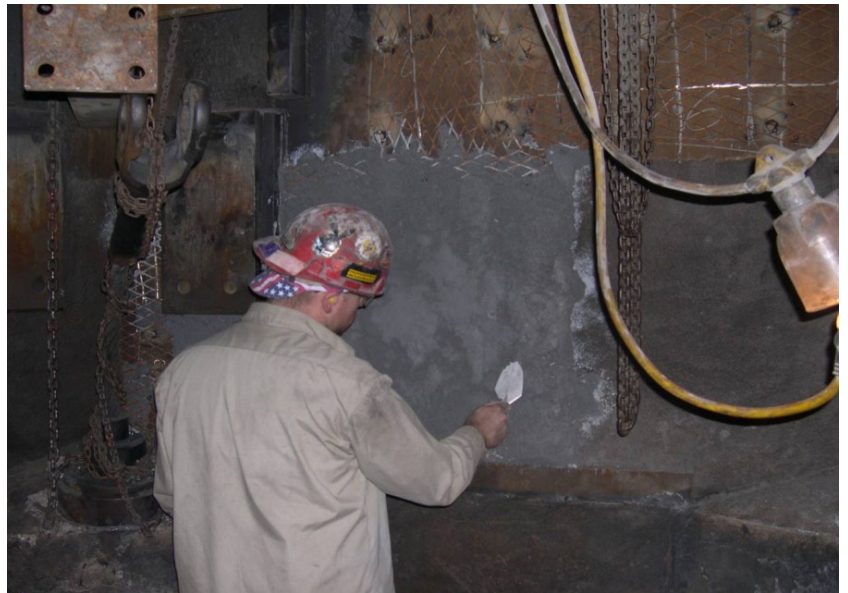
Applying Ceramite® over expanded metal mesh.
