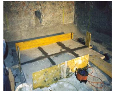
Joints are Grouted
