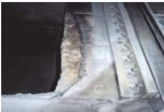
FURNACE JAMB "BEFORE"
