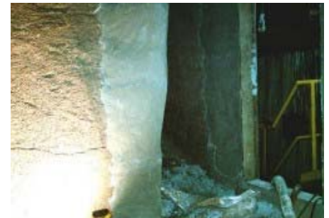
Ceramite® Trowellable retained on 1" opening 310 SS hex mesh. Solves corner and opening wear problems.
