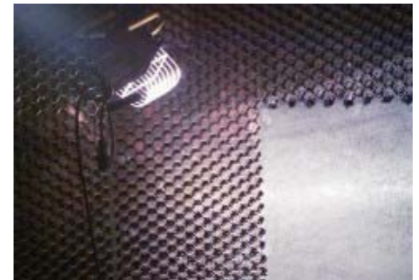
The 2" Ceramite® Trowellable lining is retained on 1" opening 310 SS hex mesh.
