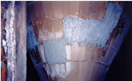
March 2003 - trowellable installed
