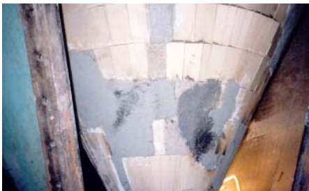
Ceramite® Trowellable installation complete - FAST, EASY, EFFECTIVE
