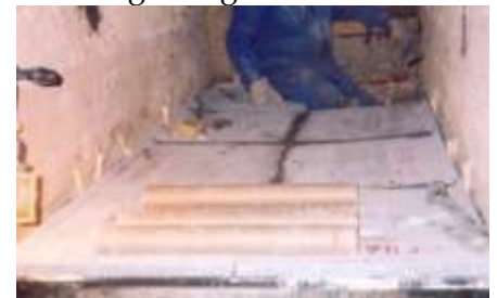
Rollers used to move tile over hearth - 8 th tile placed in these cardboard rollers.
