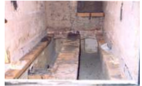
Spanner tile 2.5" low - laid in 2.5" brick for proper height.
