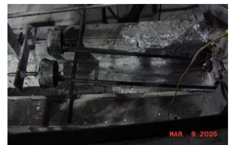
Twin Taphole Furnace
