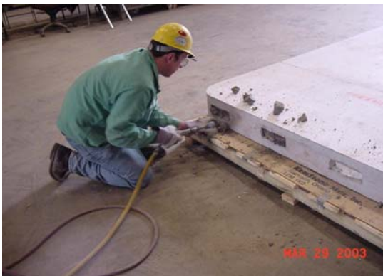
Completing Rammed Plastic Application
