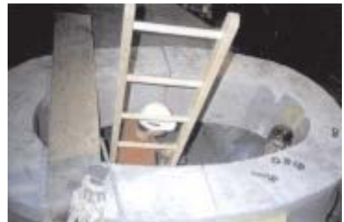
Bolting In Place
